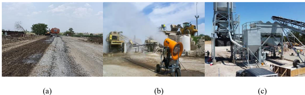
Fig. 6. Mitigation for Air Quality (a) Sprinkling water on road for dust control (b) Sprinkling water at crusher for dust control (c) Air filter at RMC plant for dust control.
